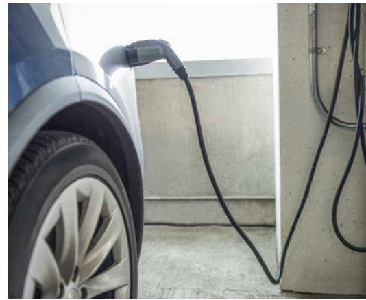
From now on the FACILITA is refueling with electricity - with help from their own innovative infrastructure for charging.
